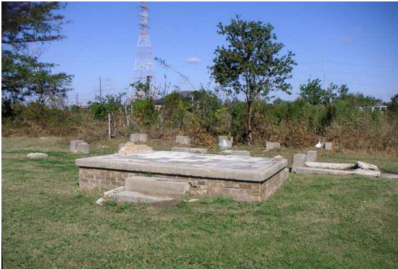
House foundation in Lower Ninth Ward.
