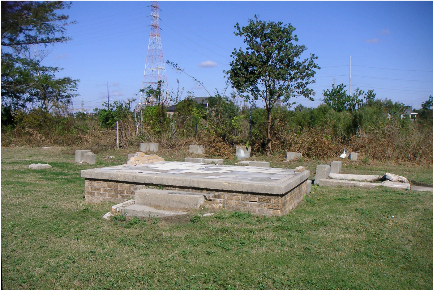
House foundation in Lower Ninth Ward.
